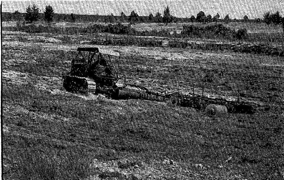
Modern procedures in scrub land development owe much to experience gained from State development of pumice lands. Rolling and discing on a State development block in the Taupo district.
